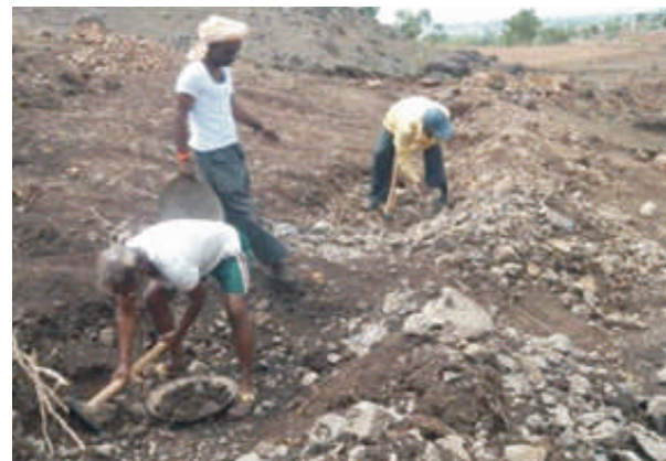
Figure 14. Constructed Contour trenching
