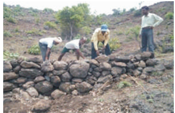
Figure 13. Constructed Gully Plugs
